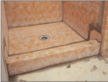
8.1 Schluter®-KERDI and 8.2 Schluter®-KERDI-DRAIN are used to waterproof a shower installation. The assembly is ready for tile setting.
